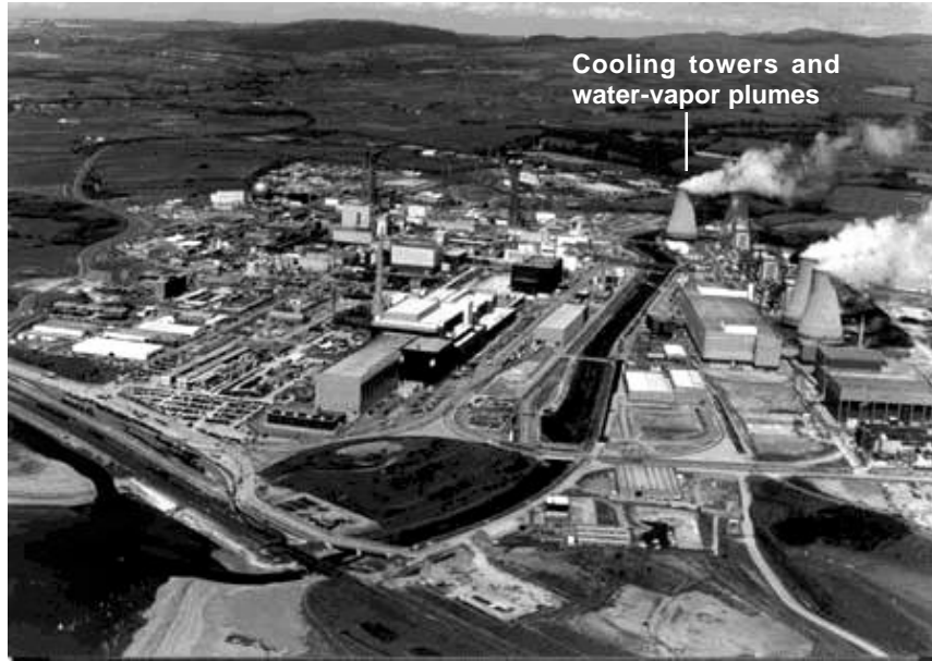
Figure 2: The four Calderhall Magnox reactors at Sellafield, United Kingdom. These four reactors made a significant contribution to the UK's plutonium for weapons. Now they have stopped producing plutonium for weapons and are producing electricity. The photograph shows the four huge natural-draft hyperbolic cooling towers of the reactors and their water-vapor plumes. Source: http://www.fas.org/nuke/guide/uk/facilit/ .
