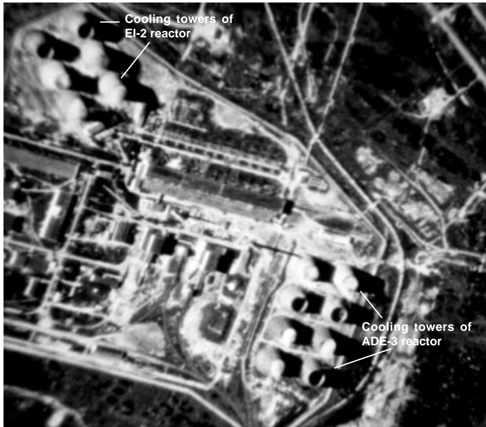
Figure 3: Declassified US CORONA satellite image of two Russian plutonium production reactors at Tomsk-7. (CORONA mission 1115-1, September 15, 1971, KH-4B with 1.8-meter resolution). The water-vapor plumes over the operating cooling towers are clearly visible.
